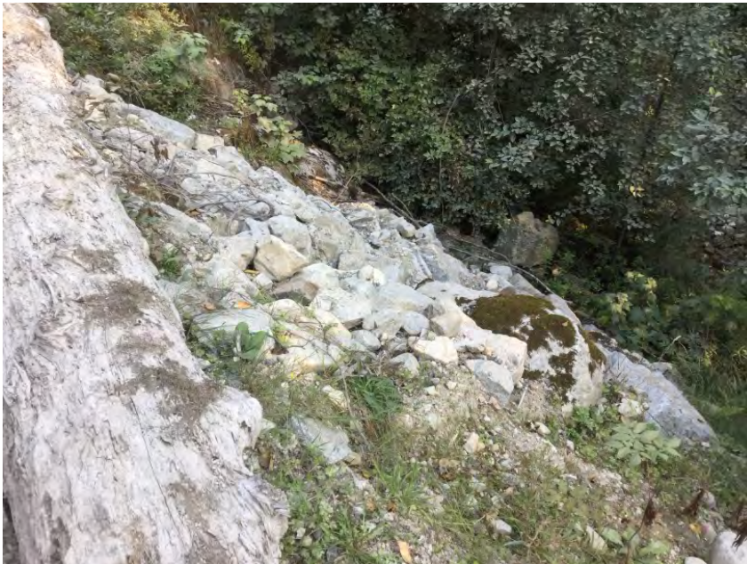
Downstream right approach fill slope repair
