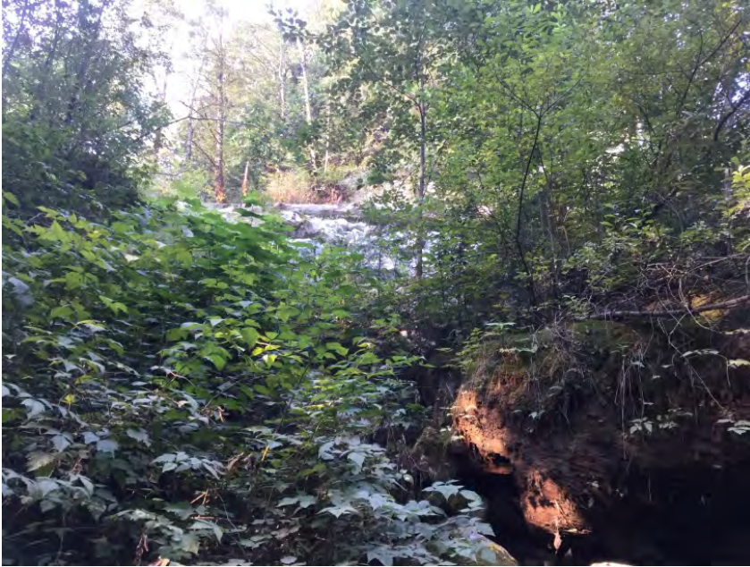
Downstream right bank fill repair immediately above large log retaining fill
